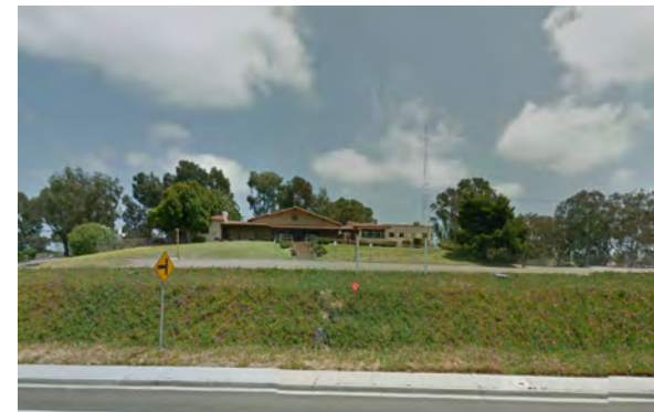
Buildings along Imperial Avenue (top) and the former Emerald Hills Golf Course (bottom) may be eligible for historic listing.
