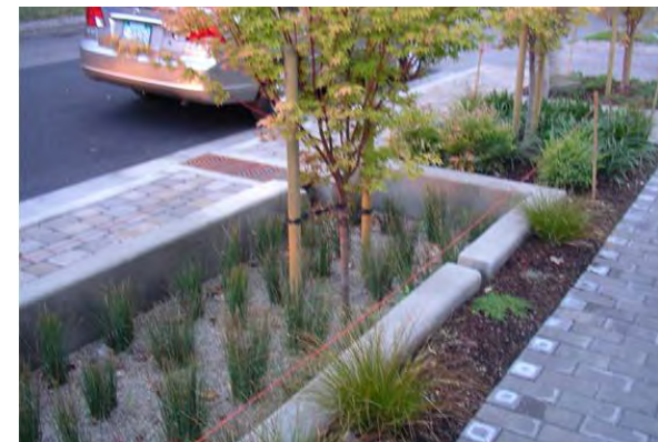
Eco-roofs, permeable paving, and bioswales are strategies to reduce solar heat gain and integrate stormwater management.
