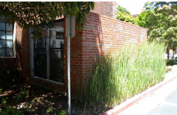
Vines and landscape should be used for screening (top). Screen all visible building equipment, utilities, and trash enclosures in a manner consistent with the building (middle and bottom).
