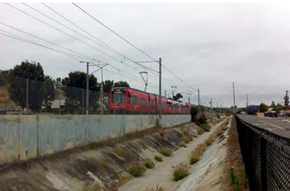
The amphitheater at Market Creek Village (top) and the path east of Euclid Avenue (middle) show the promise of creekside enhancements. Many creek segments present challenges (Imperial Avenue, bottom).
